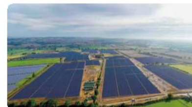
34.7MW UK's First Bifacial Dual-Glass PV Plant Yorkshire · UK Utility
