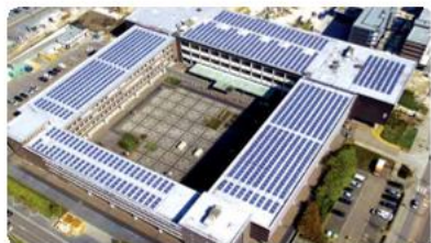
239.4KW | Genk City Hall Rooftop PV Project Genk · Belgium | Commercial and Industrial Rooftop
