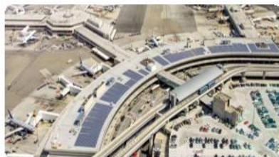
450KW | San Francisco International Airport T3 Rooftop PV Project California · USA | Commercial and Industrial Rooftop
