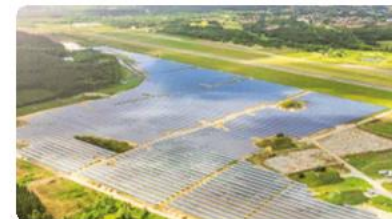
24.24MW Finow PV Plant Brandenburg · Germany Utility
