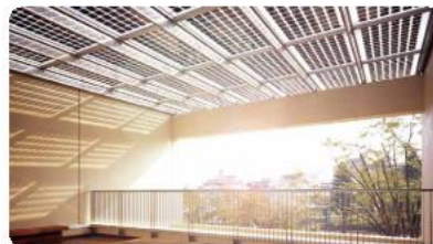
10KW | Tokyo Guanghua Primary School BIPV Project Tokyo · Japan | BIPV
