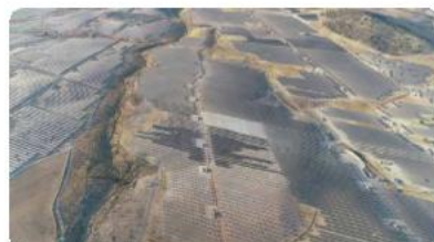
500MW (supplied 100MW) Europe's Largest PV Plant Extremadura · Spain Utility
