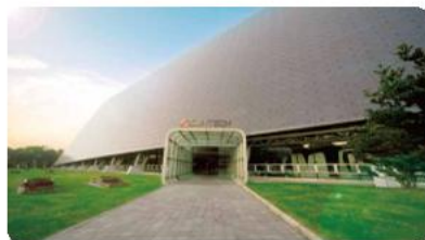
1MW | Suntech HQ BIPV Project Wuxi · China | BIPV
