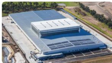
383KW | IKEA MLFU Rooftop PV Project Sydney · Australia | Commercial and Industrial Rooftop
