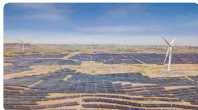
400MW Ningxia Utility PV Plant Ningxia · China Utility
